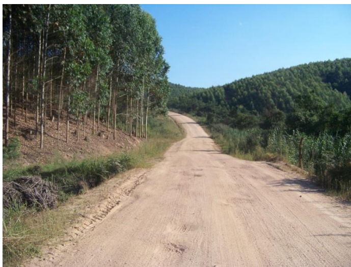
Fig 2: Deformation of road profile and formation of potholes
