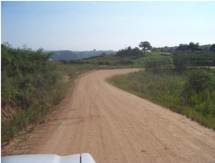
Fig. 3: Sharp bends due to mountainous terrain.
