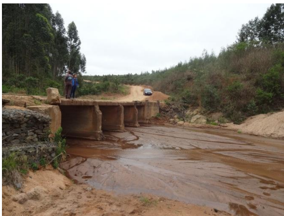
Picture 9: Existing portal culvert at km 3.0 to be upgraded.
