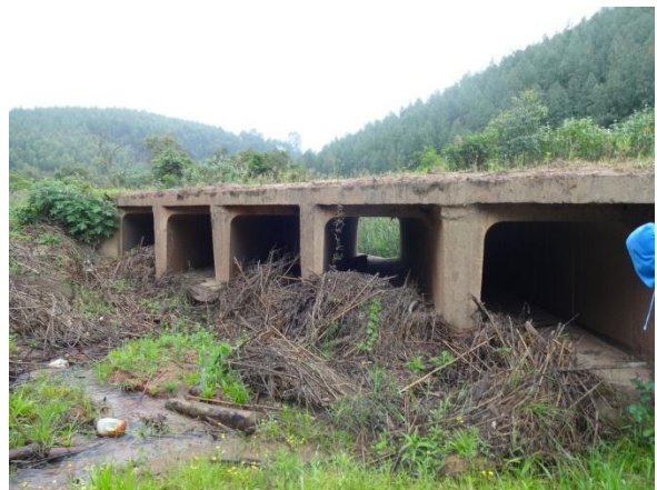
Picture 12: Existing bridge at km 7.4 to be upgraded.
