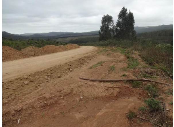
Picture 8: Taken near bend with cut off drain causing erosion to adjacent properties.
