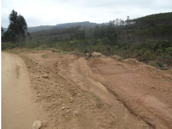
Picture 7: Taken near bend with cut off drain causing erosion to adjacent properties.
