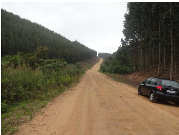
Picture 11: From km 9.0 onwards, mountainous terrain with steep sides and longitudinal slopes (valley lines) and road grades become steep to very steep passing through Eucalyptus spp.
